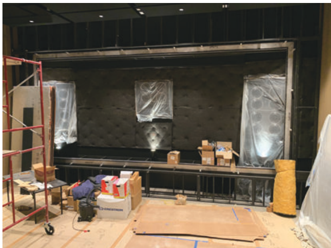
PMC LCR's mounted behind the 22-foot screen.
