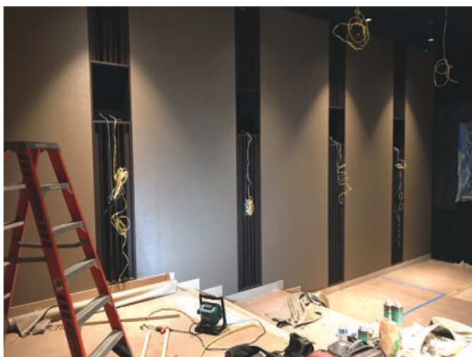
Diffusers and acoustic isolation panels on side walls.
